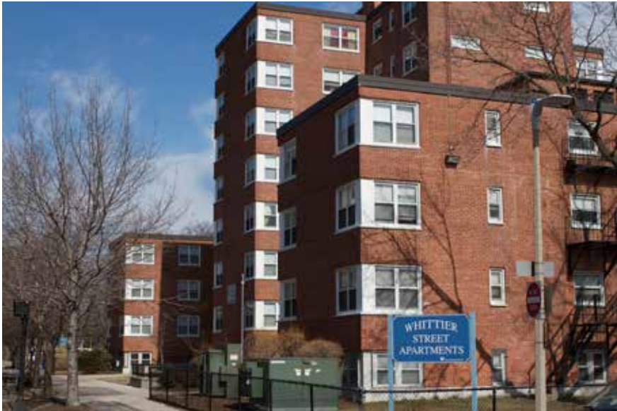
Whittier Street Apartments looking north along Tremont Street
