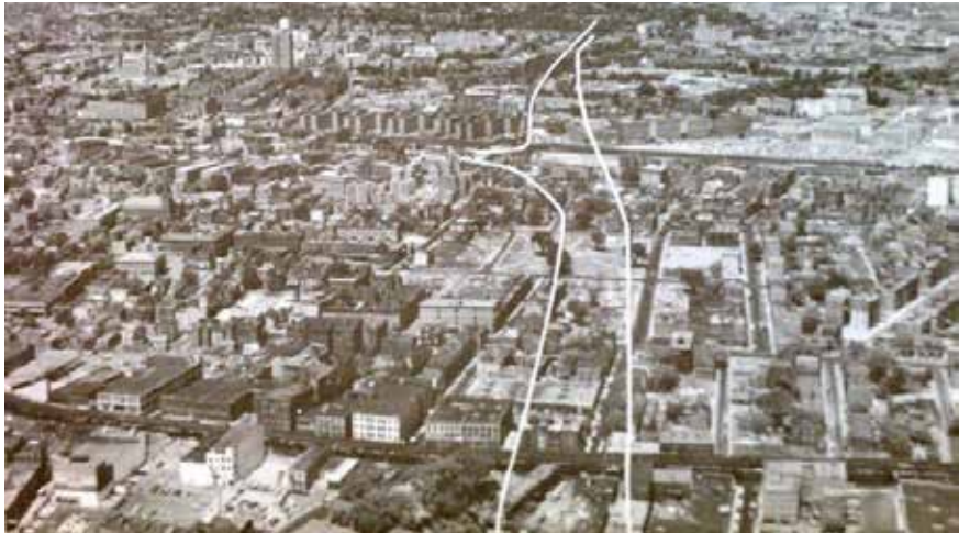
The proposed Inner Belt alignment looking east prior to demolition. Whittier Street is at the center and to the left of the proposed interchange. The right of way was cleared in the 1960s.
